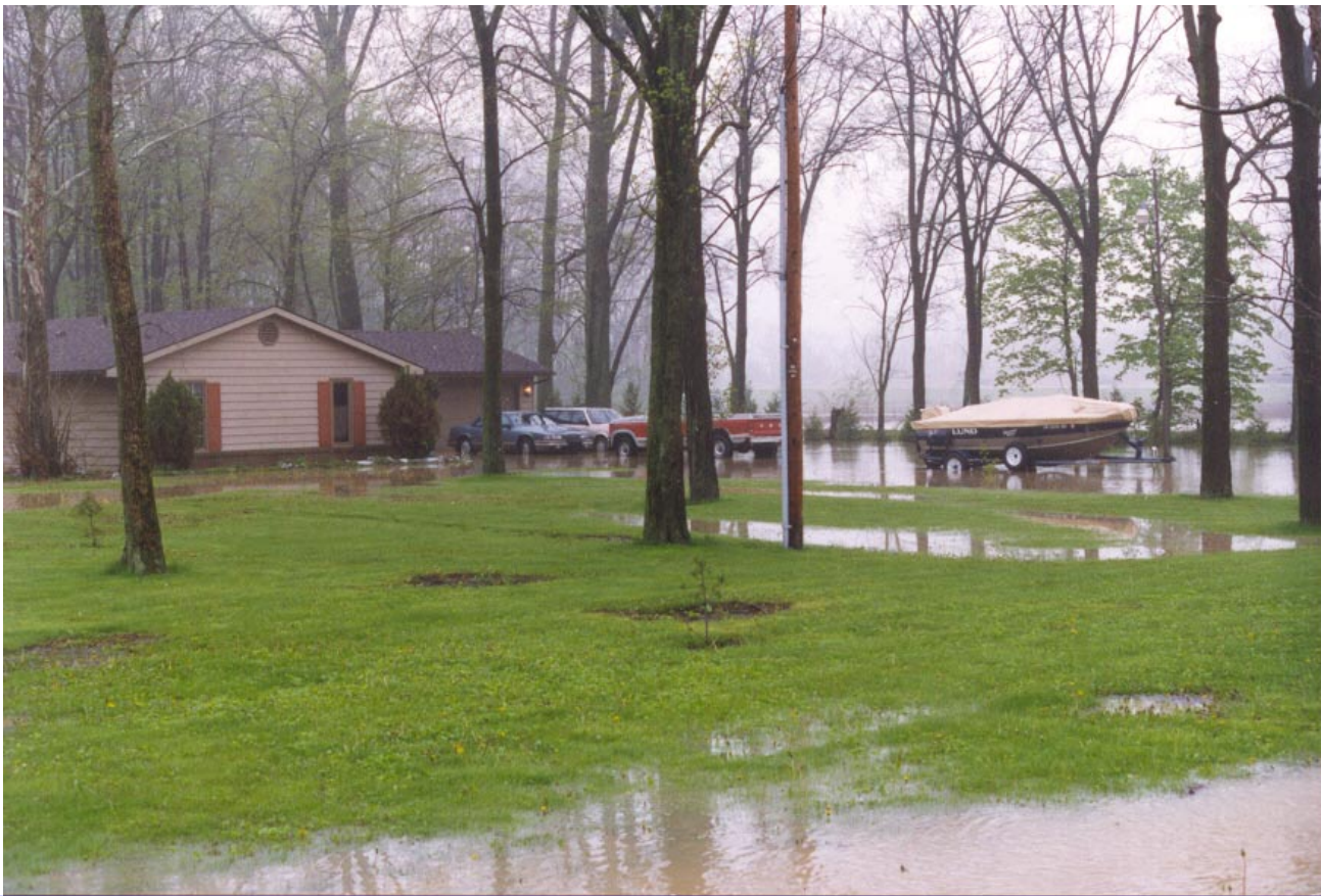
Repetitive Loss Structure with sandbags still visible. Three (3) NFIP claims filed in a ten year period. Average annual flood damages: +/- $20,000.00.
